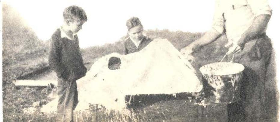
After determining the tunnel openings, dip the burlap in plaster of Paris, arrange it on the framework and build up low places with hands full of plaster as shown at left.
