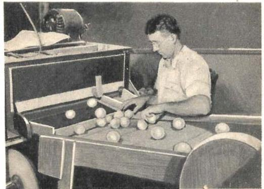
Peaches fed to a conveyor belt of this sorting machine (top) pass through a series of brushes that "shave" the fuzz off, after which peaches are selected for size and grade (bottom).
