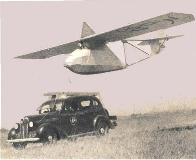
A special track mounted atop a passenger auto enables Don Stevens to launch his glider without use of tow-lines or catapults. Glider leaves auto when sufficient speed is attained. Idea inspired MM cover reproduced at right.
