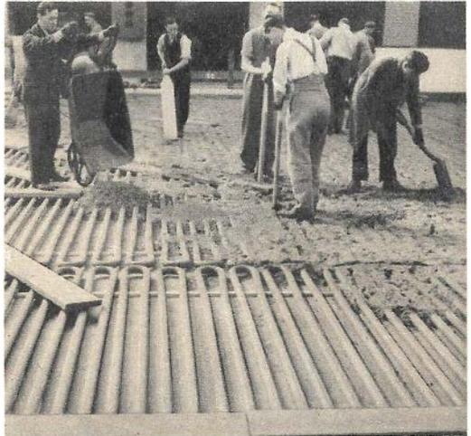
These workmen are placing packing over the nine miles of ammonia-filled piping used in making an English ice skating rink.
