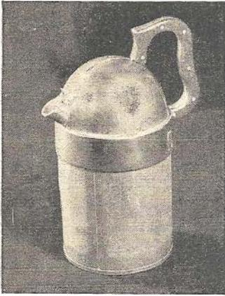
Designed to make it easier to pour milk from large sealed cans, the milk can attachment shown above consists of a metal dome featuring a movable handle that operates in a slot in the dome. The handle actuates the punch that pierces the can, making it possible to pour the milk from the can through a small spout fitted in the dome.
