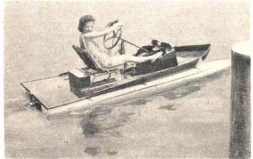
Using a 16-inch propeller, this pedal-operated boat can attain a speed of 10 m.p.h. A comfortable seat and ease of propulsion enables operator to make long trips without fatigue.
