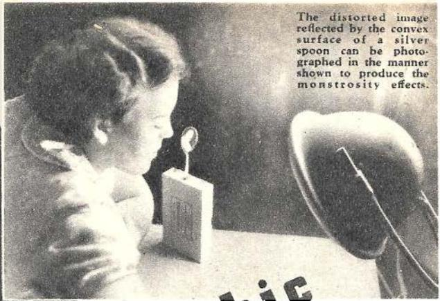
The distorted image reflected by the convex surface of a silver spoon can be photographed in the manner shown to produce the monstrosity effects.
