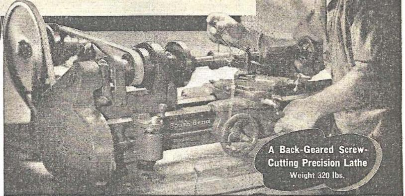
A Back-Geared Screw-Cutting Precision Lathe
