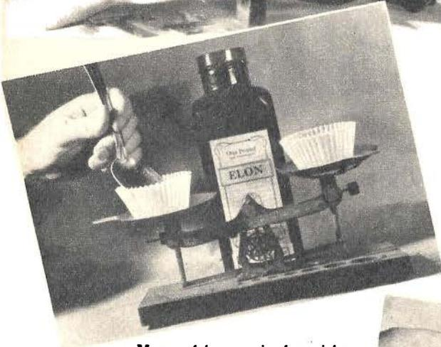
Most useful accessories for weighing up photographic chemicals are these inexpensive paper pastry cups. Due to their crinkled shape, they will hold several ounces of sulphite or carbonate without spilling. The cups insure chemical cleanliness in the darkroom.
